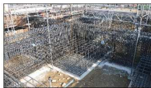
↑ [鉄筋工事の様子]
